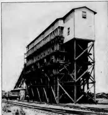
LOCOMOTIVE COALING PLANT—COAL WHARF AT ELIZABETHPORT, WITH ROBINS BELT CONVEYOR.
